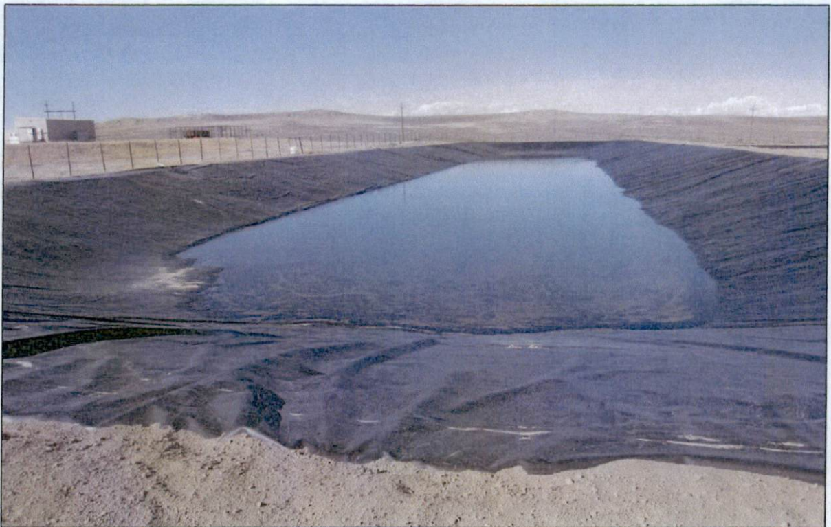
Photo #2: Completed installation of new liner in CR Pond #2.
