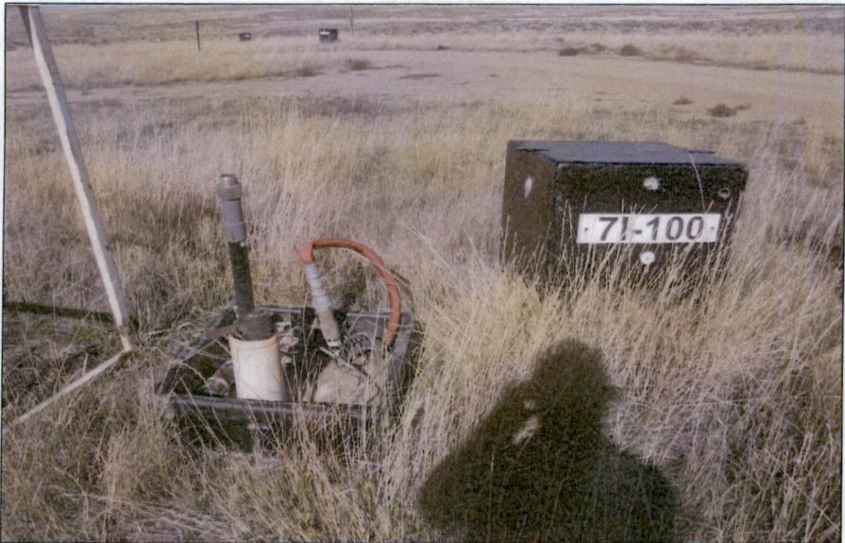
Photo #5: View of injection well converted to recovery well, stinger removed, pump installed.
