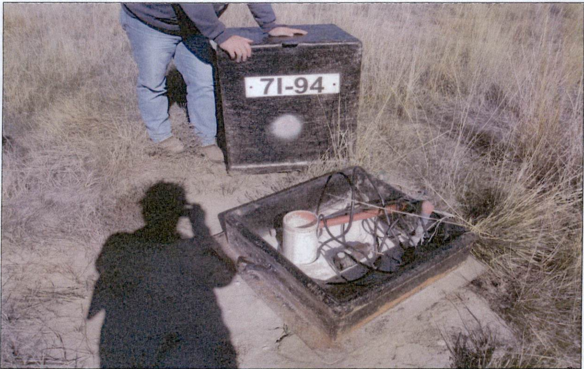
Photo #7: View of former injection well 71-94, plugged due to failed MIT.
