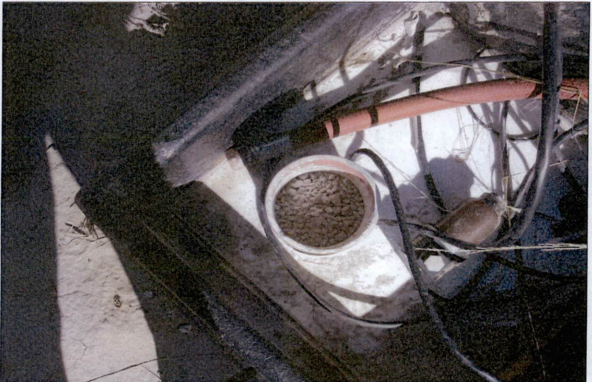
Photo #8: View of bentonite chips at surface in plugged well 71-94.
