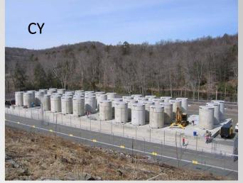
15 Spent Fuel Dry Casks 1 GTCC Dry Casks NAC MPC System CoC Expires 4/10/20
