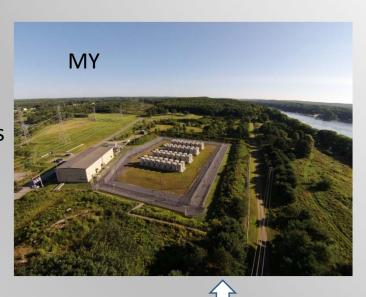
40 Spent Fuel Dry Casks 3 GTCC Dry Casks NAC MPC System CoC Expires 4/10/20
