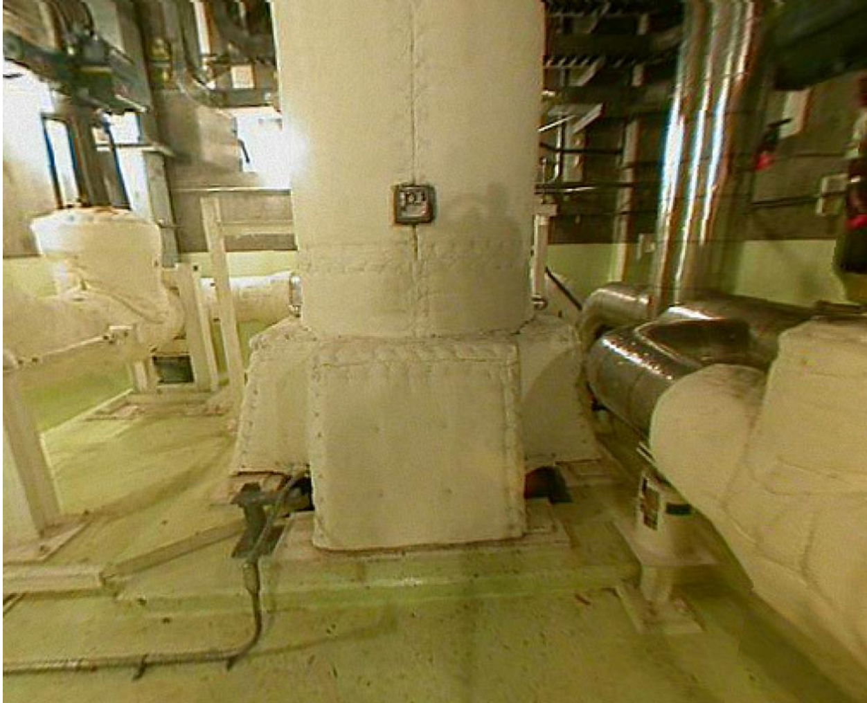
Figure 3ISI-19.2 Photograph of RHR heat exchanger S-1 supports with insulation. The Insulation is removed for surface examinations.
