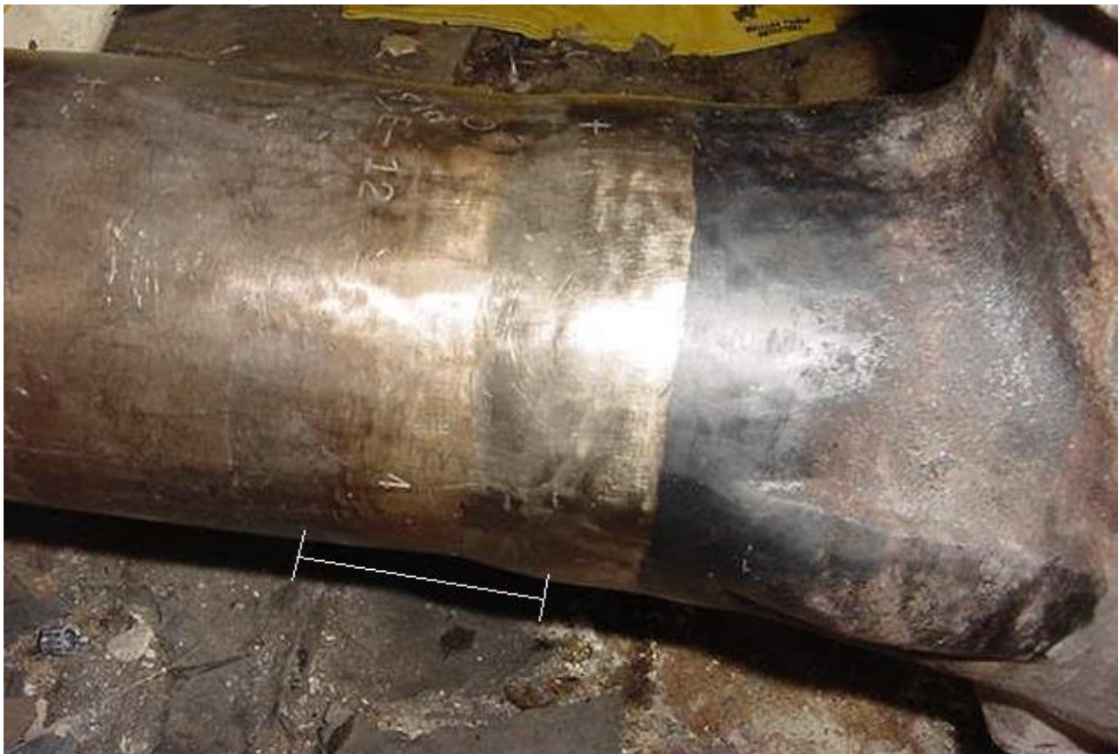
Figure 3ISI-17.2 Photograph of weld 4RRC(4)B-12 highlighting the mismatch in the transition area from the pipe to the valve taper.
