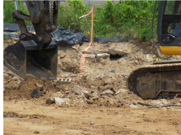
Figures 9 and 10 Examples of Debris that was Exhumed During Remediation Excavation of the Burial Pit Area
