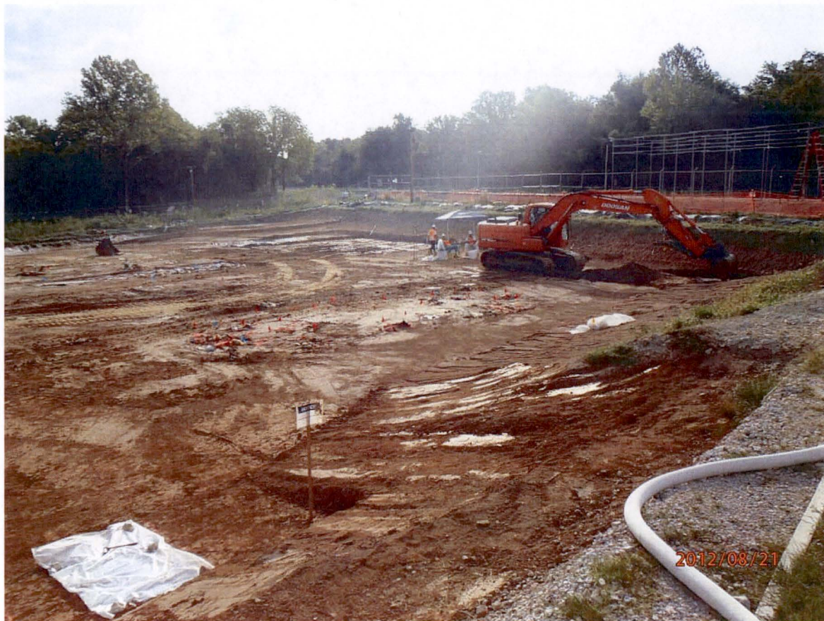
Figure 3-2 Burial Pit Becoming Clearly Visible after Overburden Removal (LSA 10-14)
