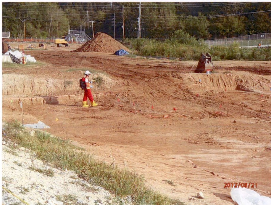
Figure 3-1 Early Stage of Remedial Excavation in South Burial Pit Area (2012)
