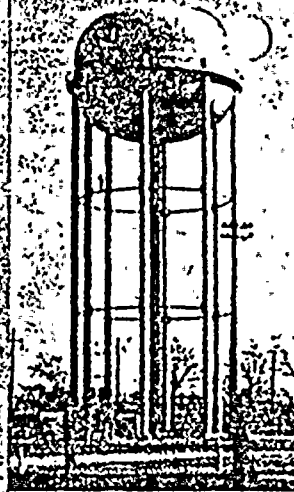
TANKS: Cold galvanized with Z.R.C. in 1964 — still good for several years (Galena, Park, Texas)
