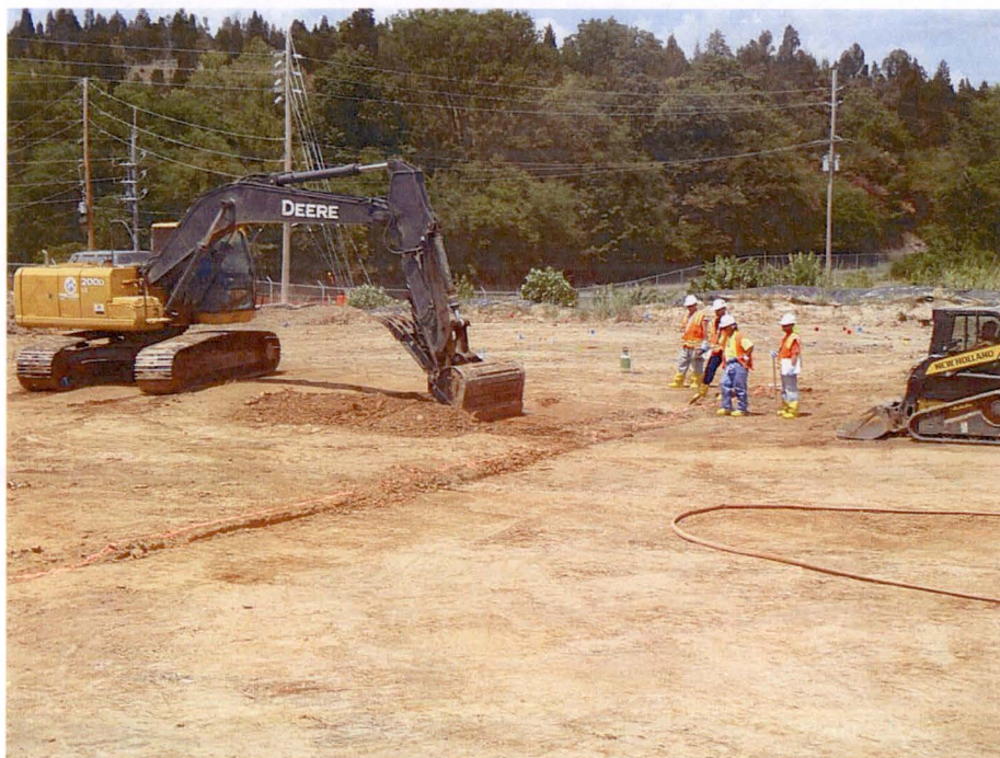
Figure 3-1 Early Stage of Remedial Excavation in Burial Pit Area (2012)
