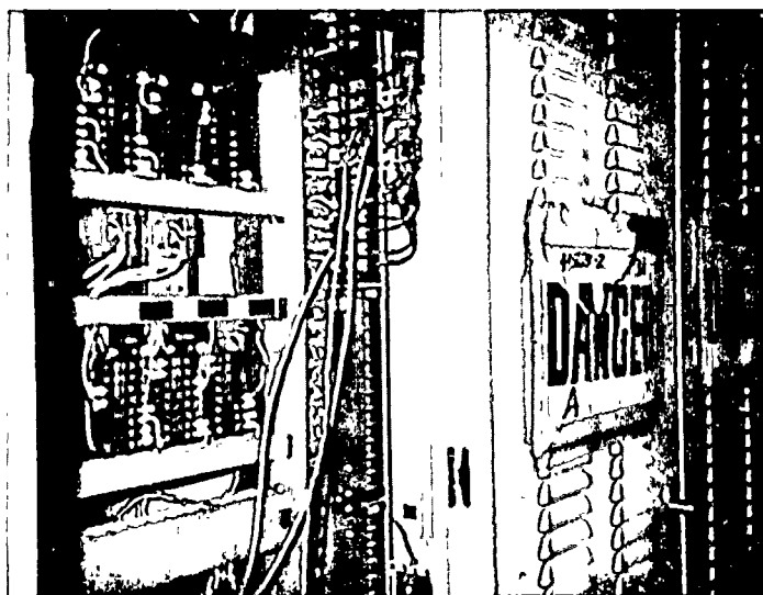
PHOTO #4 TEST SET-UP RACK #12 REAR VIEW BISTABLE MONITORING CONNECTIONS
