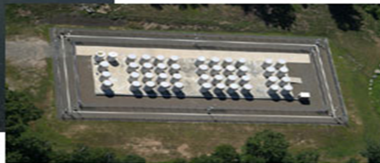
Below: The CY Independent Spent Fuel Storage Installation.
