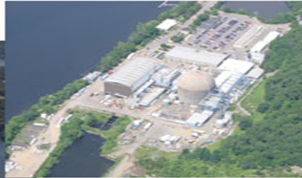
Above: The Connecticut Yankee site in 2003, before structural demolition.
