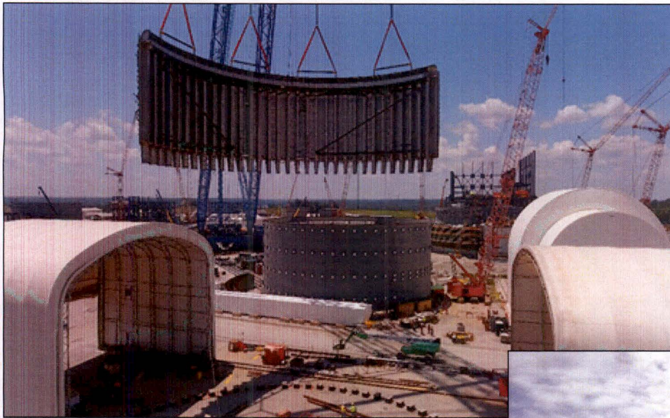
Placement of the In-containment refueling water storage module, VC Summer Unit 2
