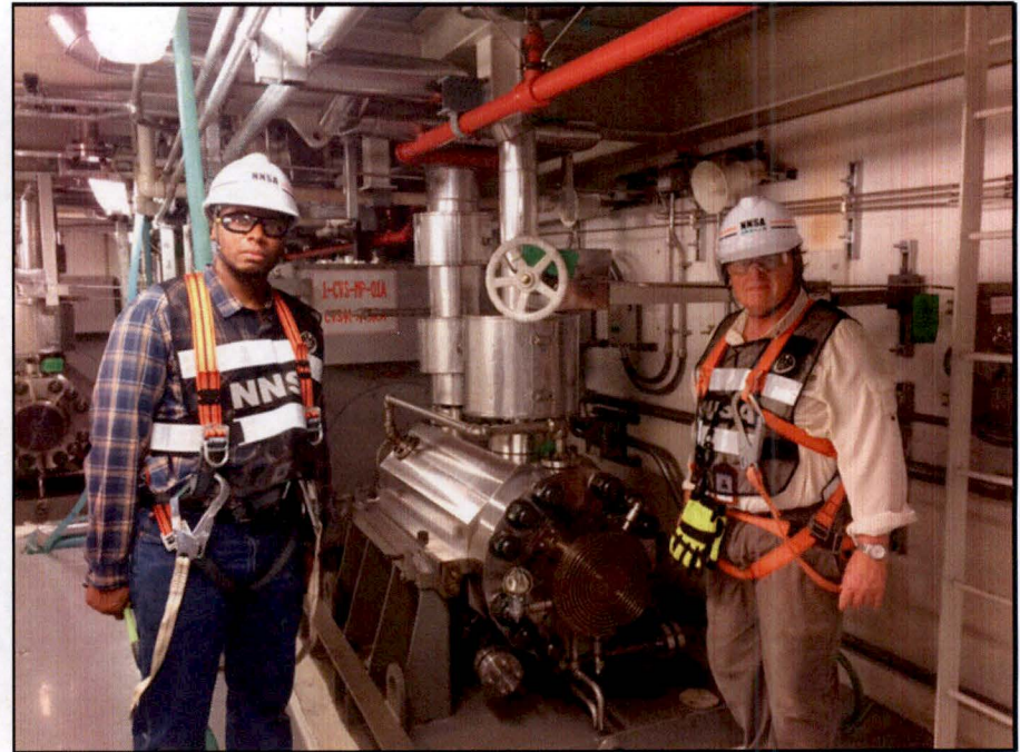
Chemical and volume control system pumps
