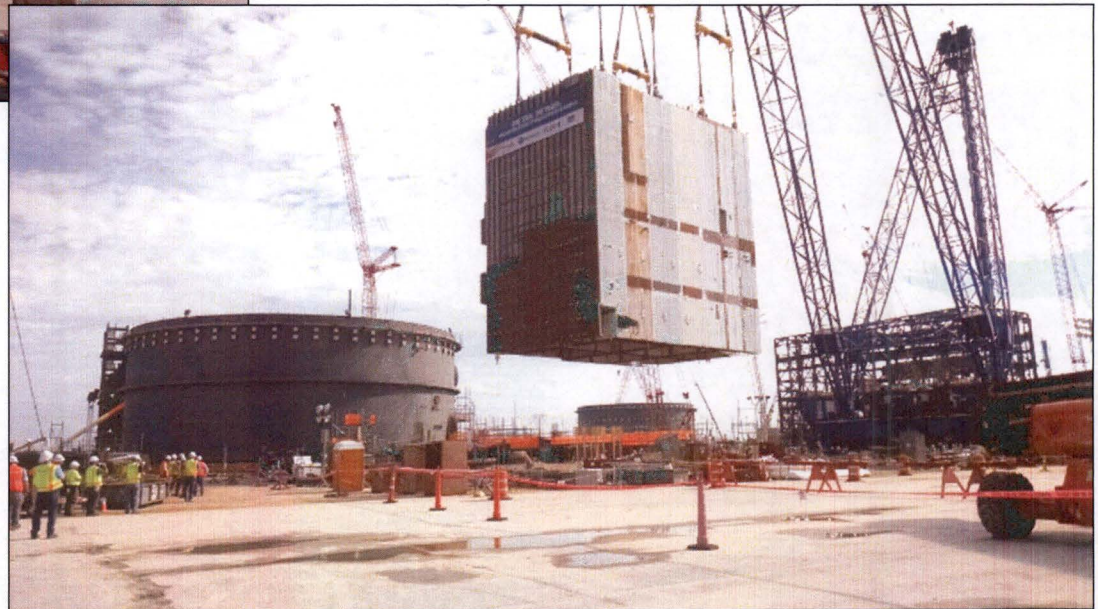
Placement of the Auxiliary Building Module, Vogtle Unit 4
