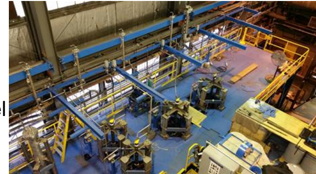
Mechanisms Engineering (Sodium) Test Loop at ANL
