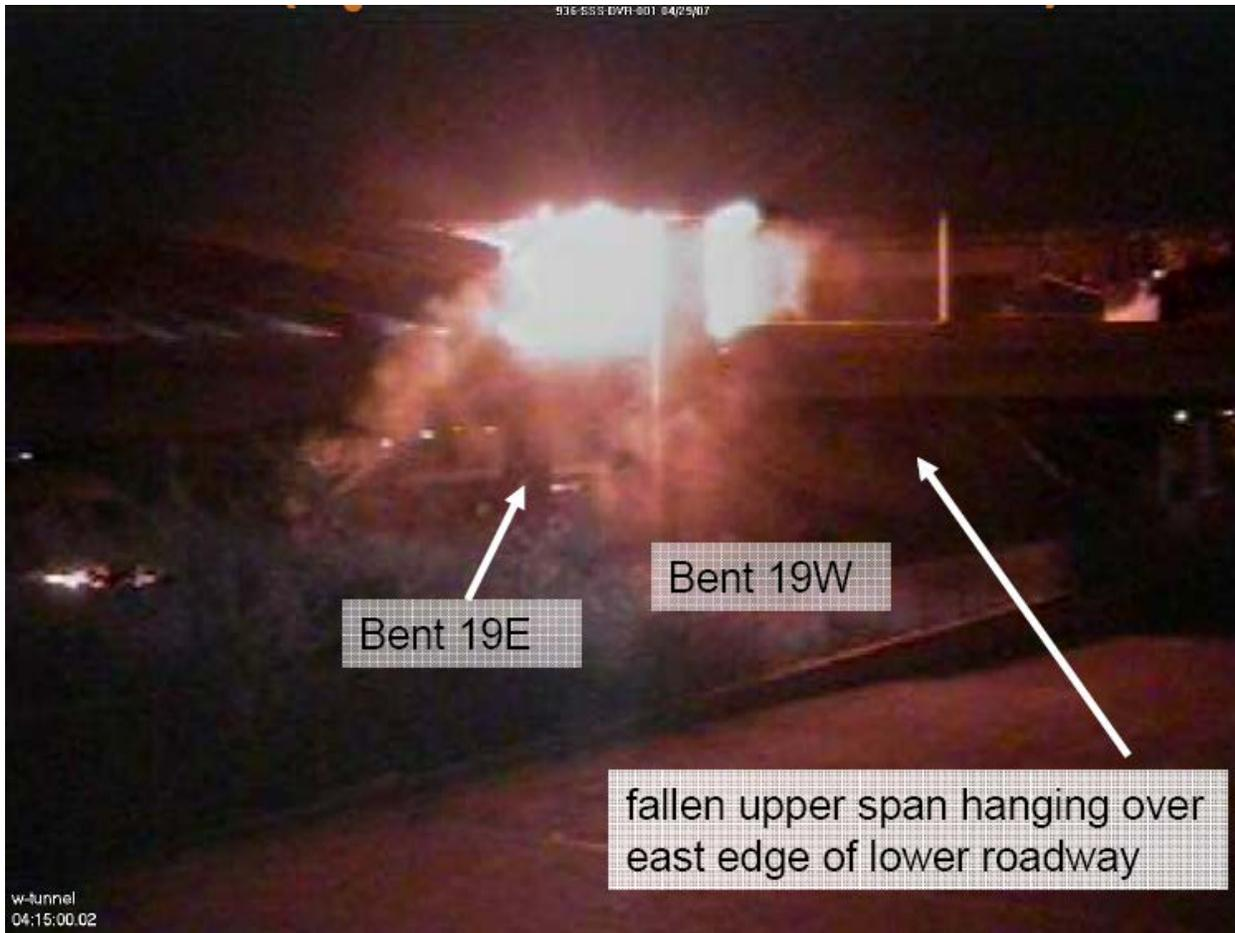
Figure 2.5. MacArthur Maze Fire at +37.3 Minutes (WTP video image at 04:15:00.02 PDT, photo from MAIT Report, CHP 2007, reprinted with permission.)
