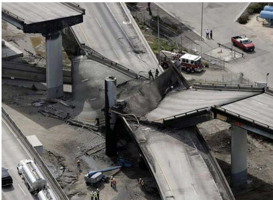
Figure 1.1. Roadway Configuration after the MacArthur Maze Fire (photo from MAIT Report, CHP 2007, reprinted with permission.)
