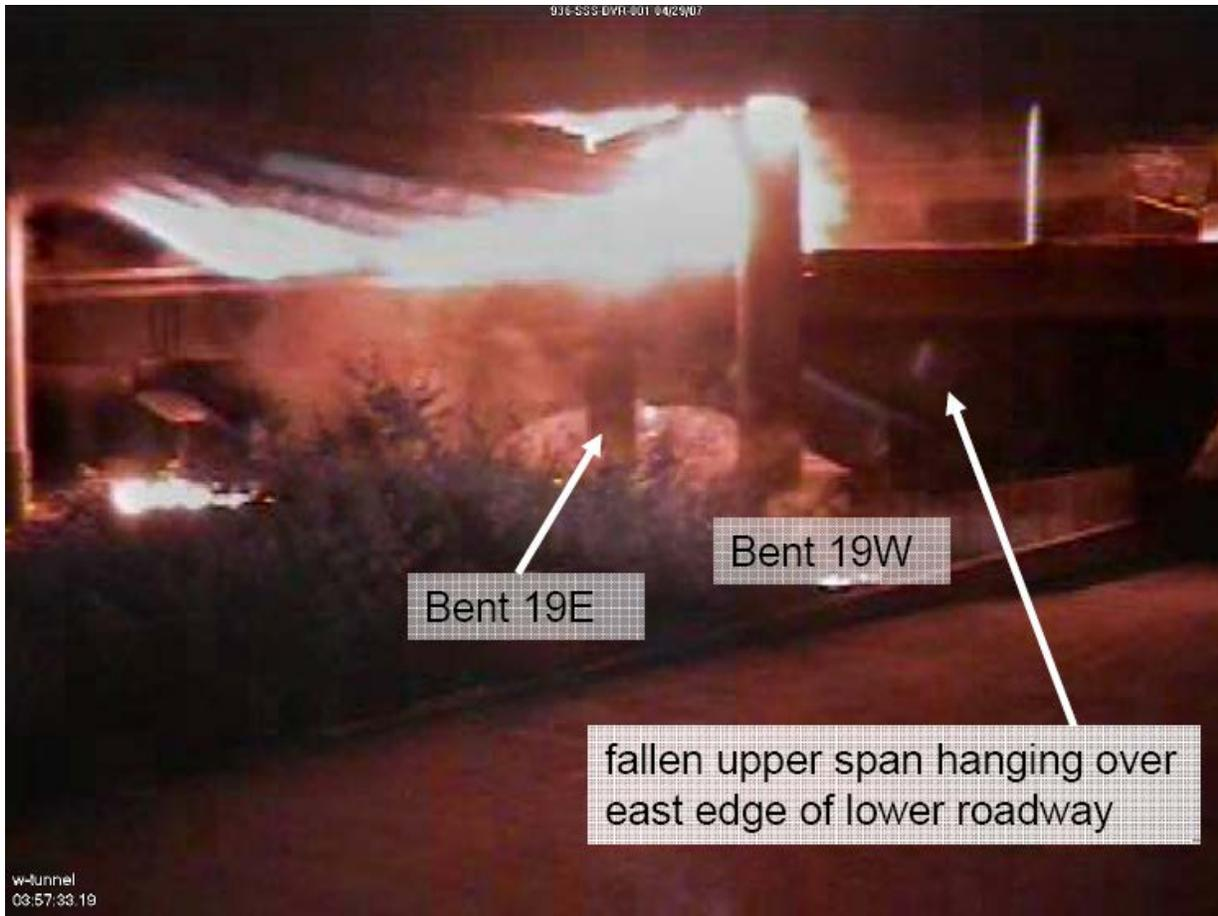
Figure 2.4. MacArthur Maze Fire at +19.8 Minutes (WTP video image at 03:57:33.19 PDT, photo from MAIT Report, CHP 2007, reprinted with permission.)
