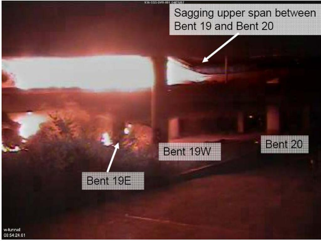
Figure S.1. MacArthur Maze Fire at +16.7 Minutes (WTP Video Image at 03:54:24.61 PDT, photo from MAIT Report, CHP 2007, reprinted with permission.)
