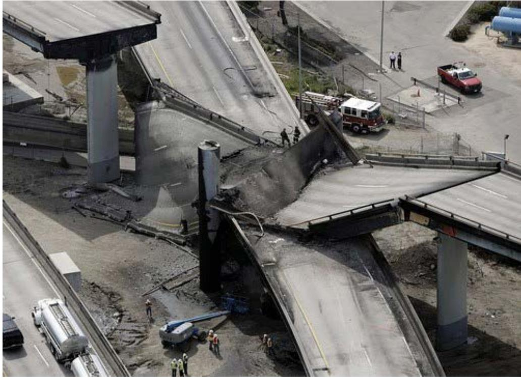
Figure S.2. Roadway Configuration after the MacArthur Maze Fire (photo from MAIT Report, CHP 2007, reprinted with permission.)
