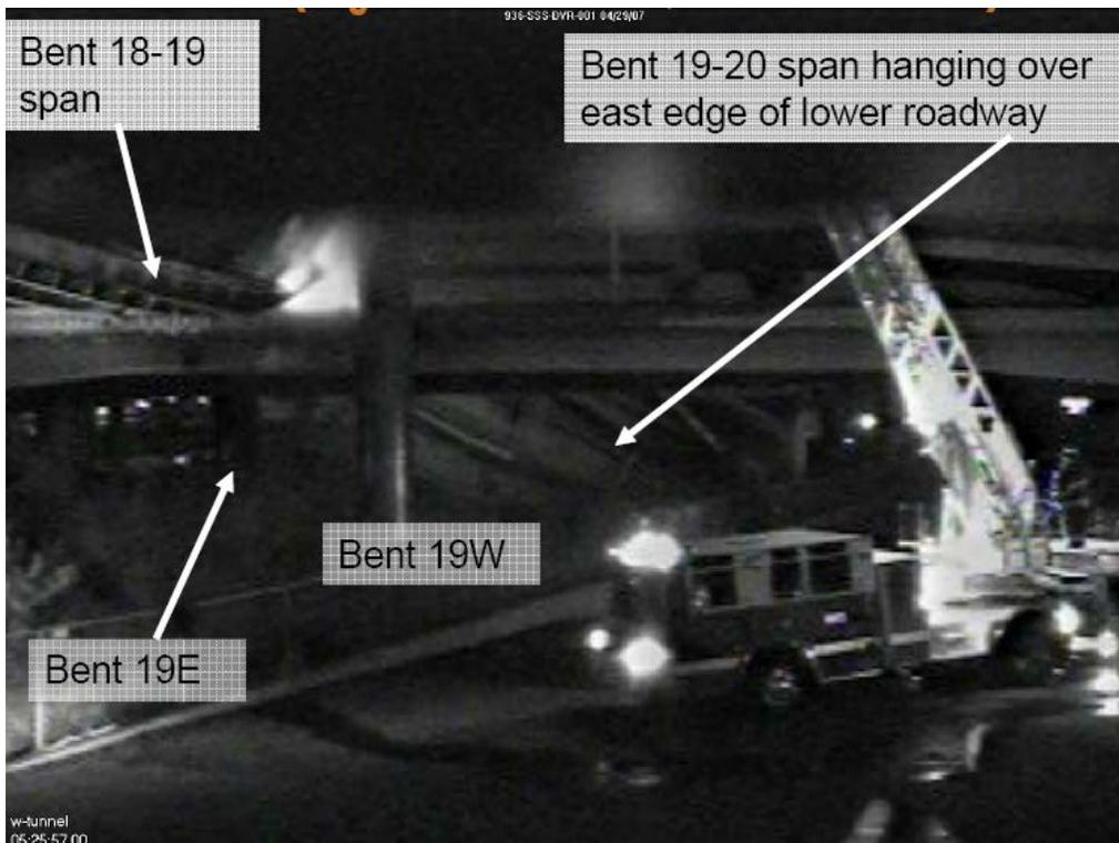
Figure 2.7. MacArthur Maze Fire at +107.3 Minutes (WTP video image at 05:25:57.00 PDT, photo from MAIT Report, CHP 2007, reprinted with permission.)
