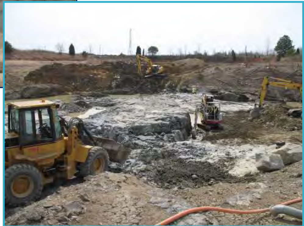
Existing Lee Unit 2 Excavation Cleanup
