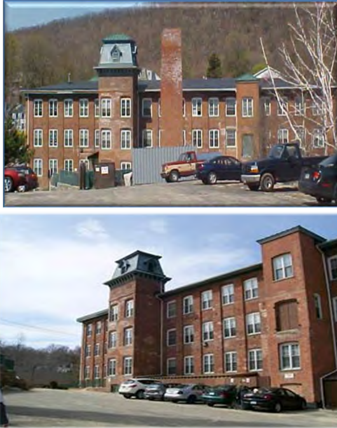
Figure 3. 13 Wallens Street (Gilbert Clock Shop Apartments in 2009) (Google Earth, 2015)
