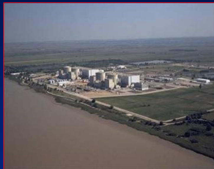
E. De Fraguier, "Lessons learned from 1999 Blayais flood: overview of EDF flood risk management plan," U.S. NRC Regulatory Information Conference, March 11, 2010.
