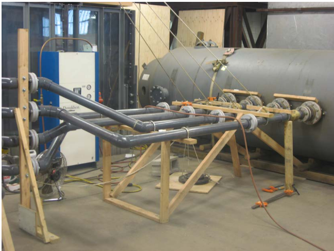
Figure 3. Additional photographs of the steam delivery system at nominal one-eighth scale. (Ref. 1)
