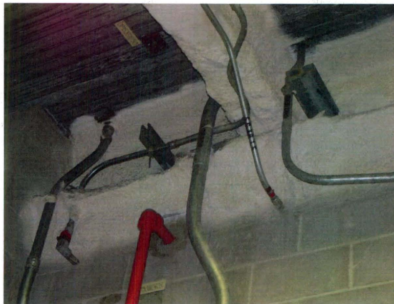
Figure 12.2.2-2 Typical Fireproofed Steel Integral to a Fire Barrier
