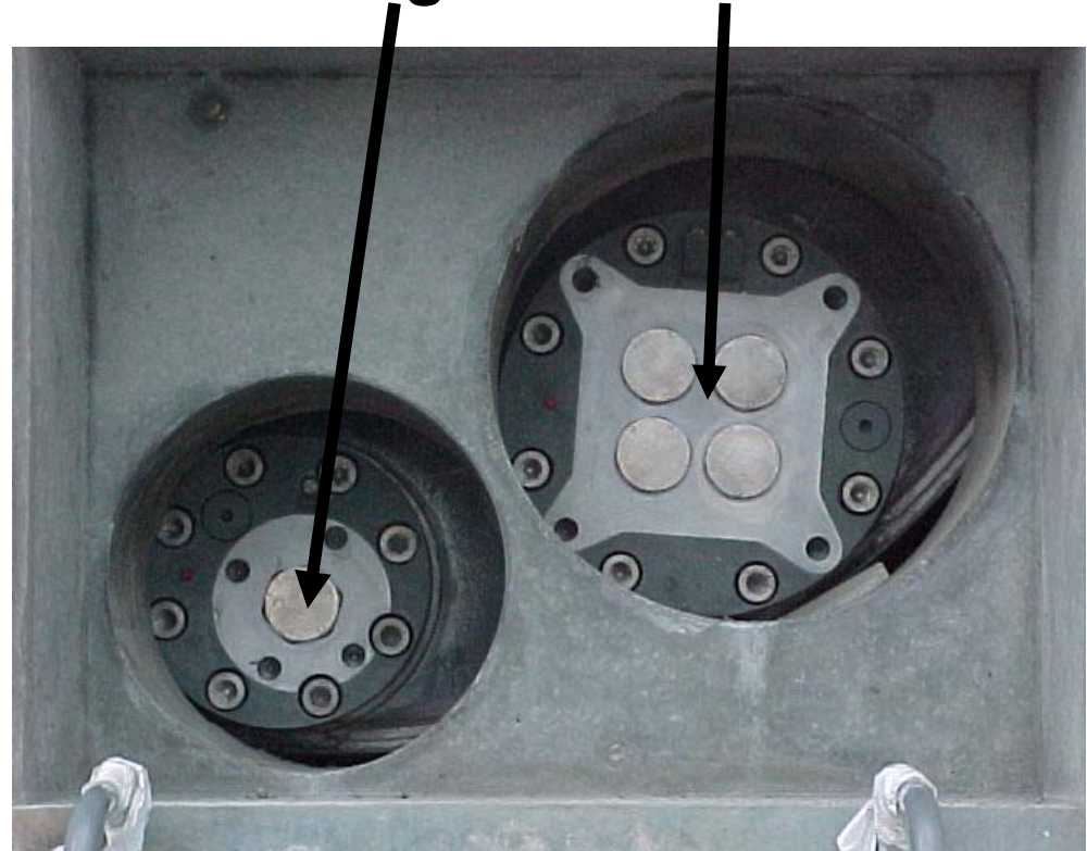
View via HSM Rear Access Door
