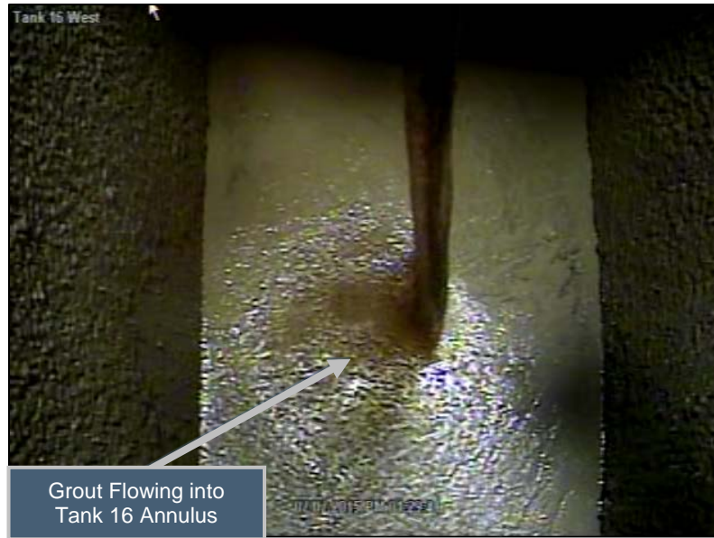
Figure 3.2-6: Annulus Bulk Fill Grout during the Filling Process (Lift 4)
