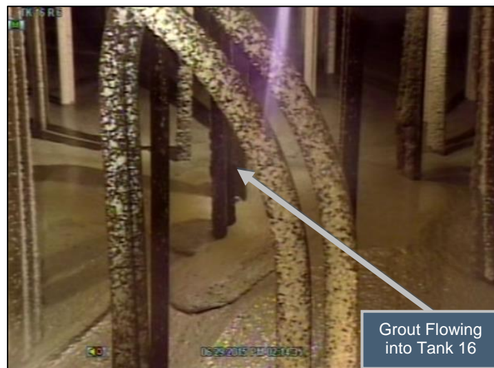
Figure 3.2-2: Bulk Fill Grout during the Filling Process (Lift 3)
