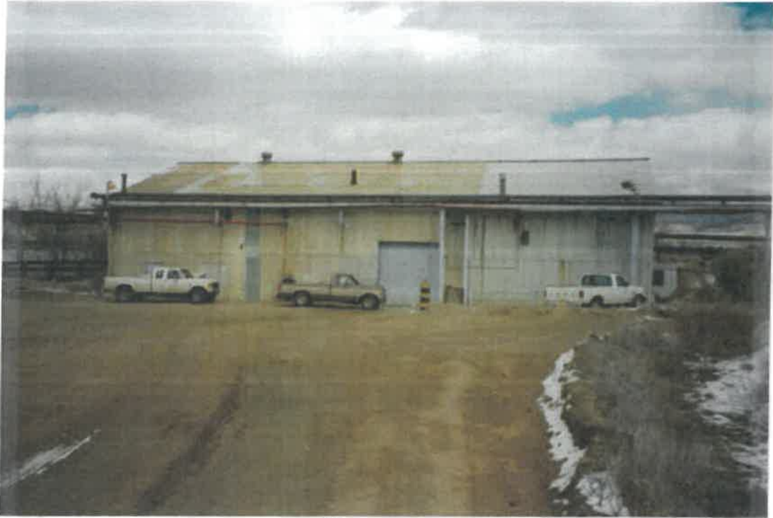
Photograph 3 - IX Plant Building, Currently in Use.
