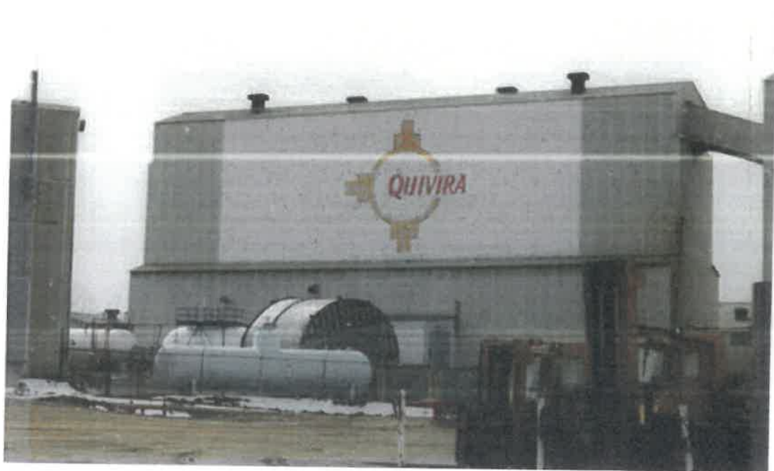
Photograph 2 - Site Logo on Conventional Mill Building.
