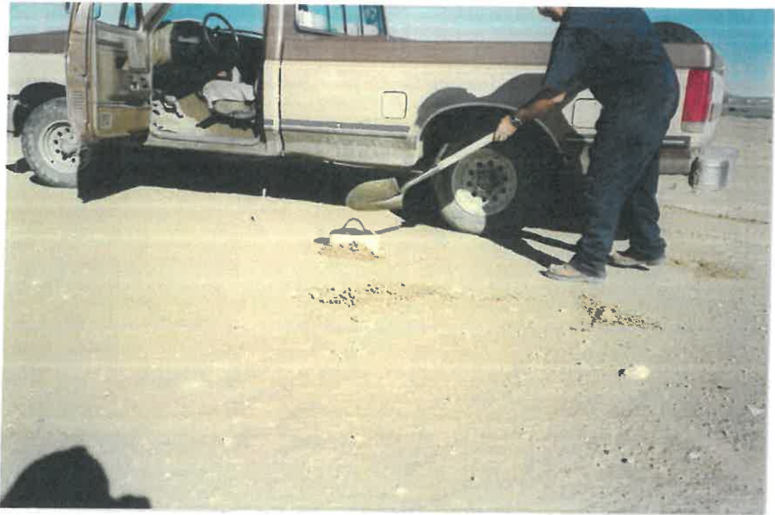
Photograph 5 - LAACC being installed on Pond 2.
