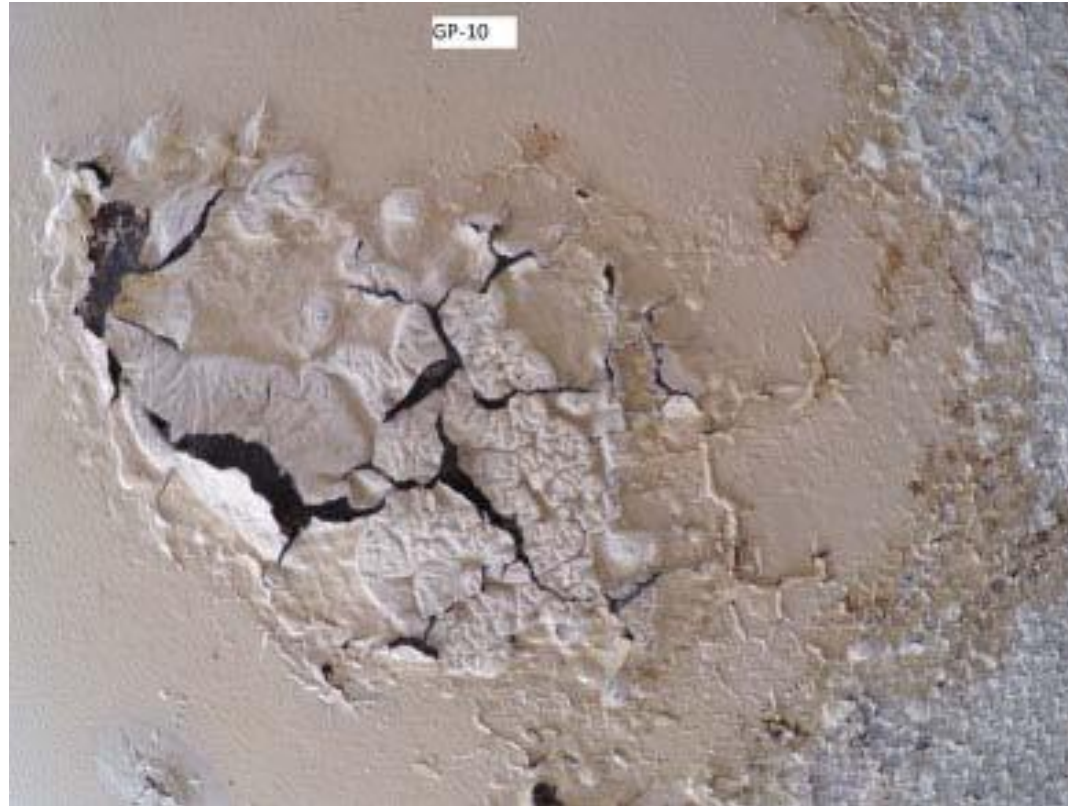
GP-10 showing no detectable loss of material from base metal
