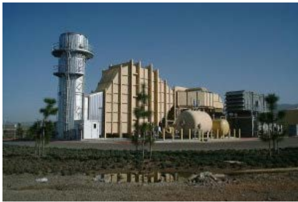
Simple-Cycle, 260 MW
