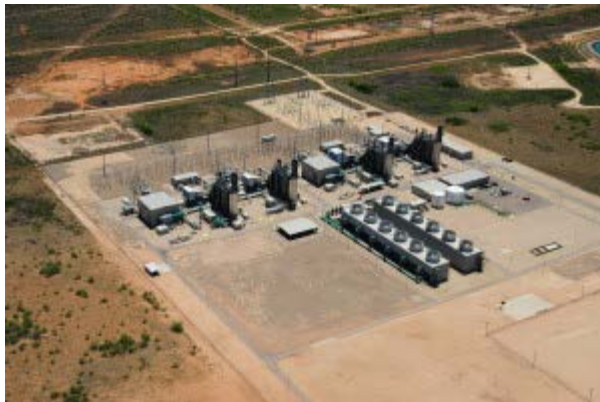
Combined-Cycle, Natural Gas-Fired Plant, 550 MW
