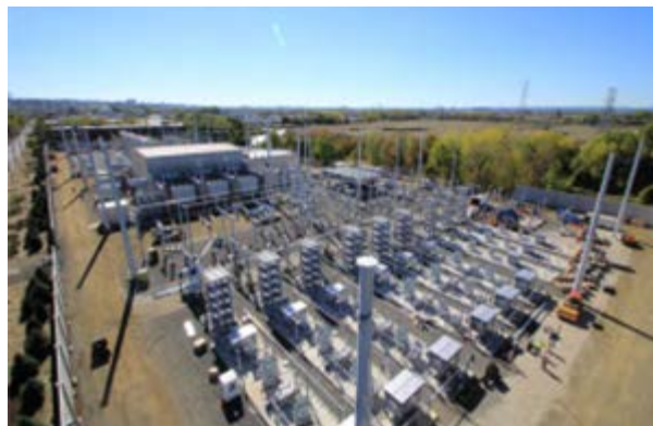
Underground / Sub-sea Trans, 660 MW
