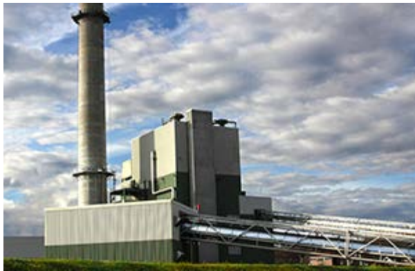
Wood Biomass-Fired Power Plant, 75 MW
