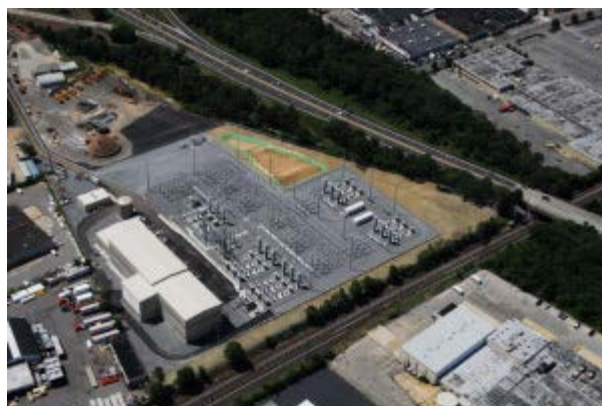
High Voltage DC Transmission, 660 MW
