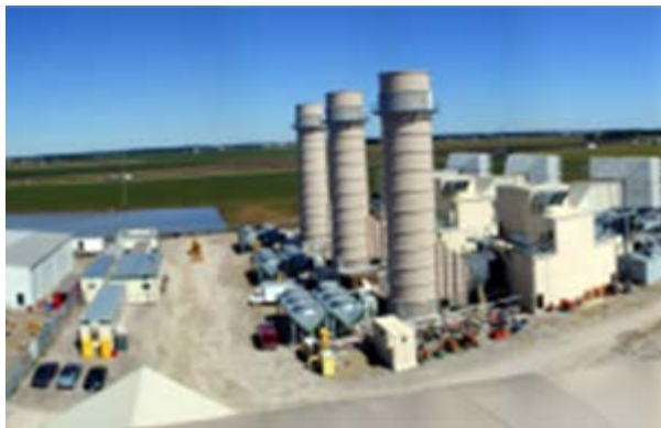
Simple-Cycle, Natural Gas-Fired Peakers, 444 MW (Richland), 20 MW (Stryker)
