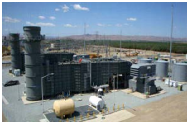
Simple-Cycle, Natural Gas-Fired Peaker, 120 MW
