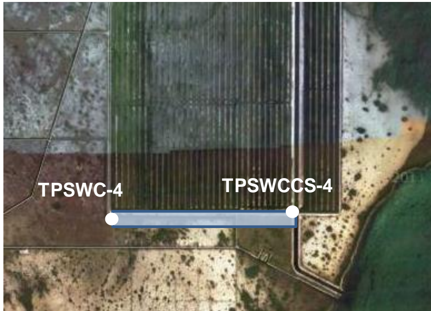
Figure 5.4-4. Locations of TPSWCCS-4 and TPSWC-4 Monitoring Stations; Conceptualized Seepage from Southern Collector Canal into the CCS is Shown.
