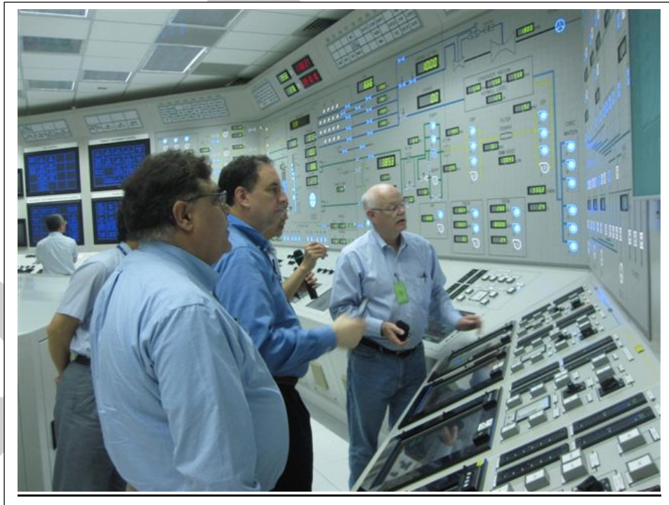
NRC staff tour an all-digital control room at the Taiwan Electric Company Lungmen Nuclear Plant in 2010
