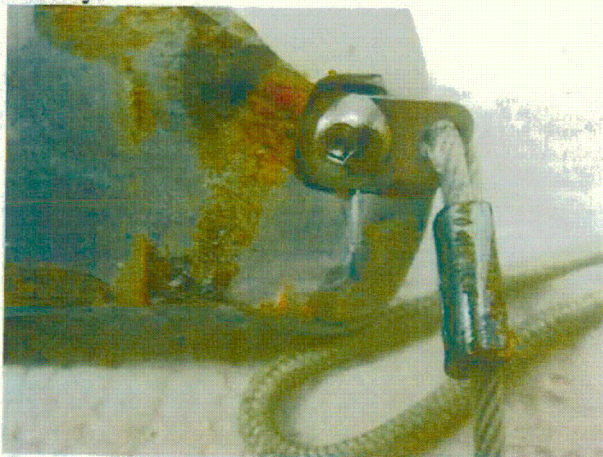
Lock Cover assembly with crack at screw
