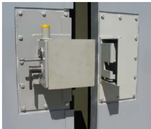
Figure 4. Internal locking device
