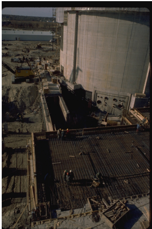
figure 5 Foundation Penetrations 1973 Zion Station Construction Photographs Zion, Illinois
