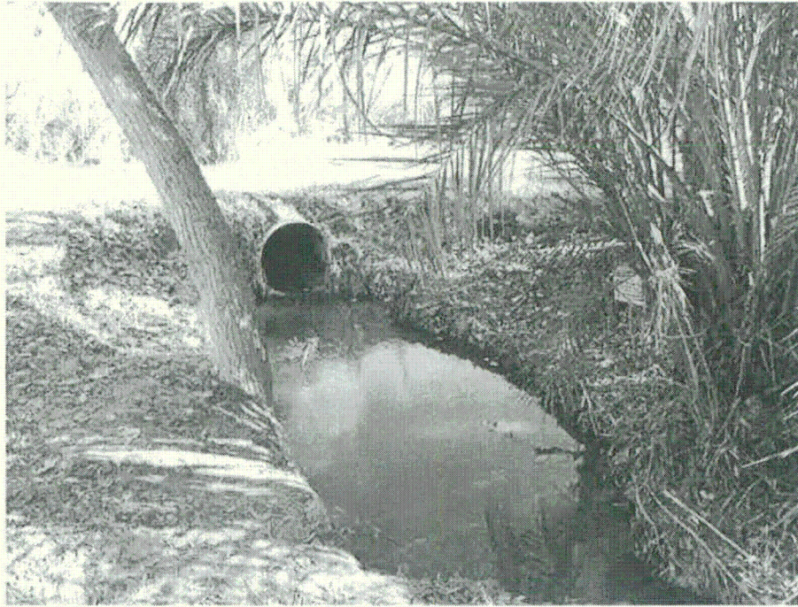
Photograph 3: Downstream flow of spring water within China Ranch property
