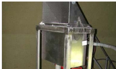
Passive autocatalytic recombiners
