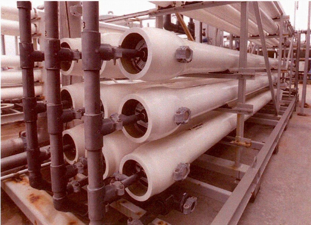
Diablo Canyon Power Plant's desalination filters are shown in this photograph. San Luis Obispo County and Pacific Gas & Electric Co. are working together to explore the possibility of utilizing the plant's excess water as a supplemental source for the county.
