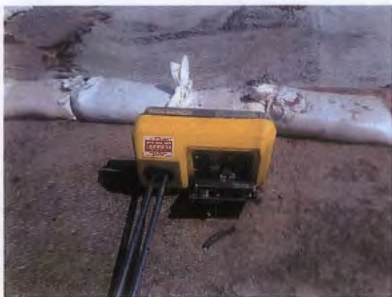
Gauge – Closeup of cover plate
