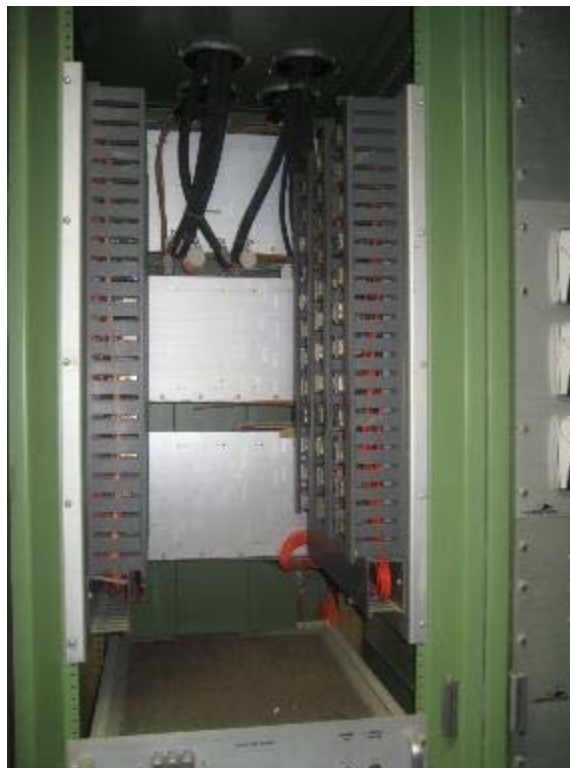
Figure 4-6 An Example of Non-Enclosed Wire-Ways That Would Not Qualify as Metal Enclosed Wire-Ways
