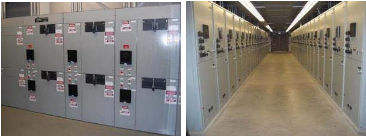
Figure C-1 Front View of Medium Voltage Switchgear Banks
