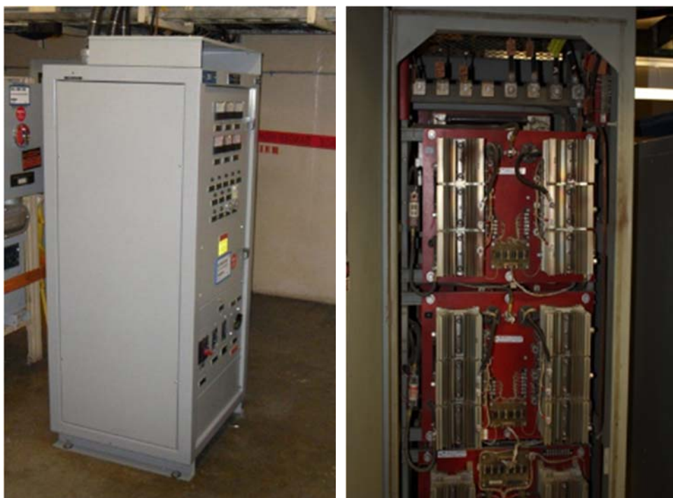
Figure 3-5 A Typical Inverter Cabinet (Exterior – Left, Interior – Right)
