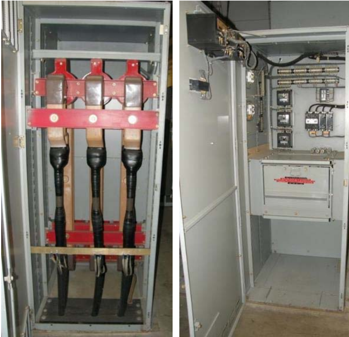
Figure C-4 Internal Views of Medium Voltage Switchgear, Back Showing Bus Cables (Left), Front Showing Control and Relay Enclosure (Right)
