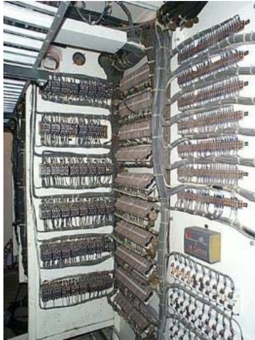
Figure C-20 Large Open Electrical Enclosure (Walkthrough Enclosure)
