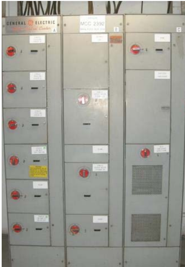
Figure C-11 Front View of MCC with Three Vertical Sections
