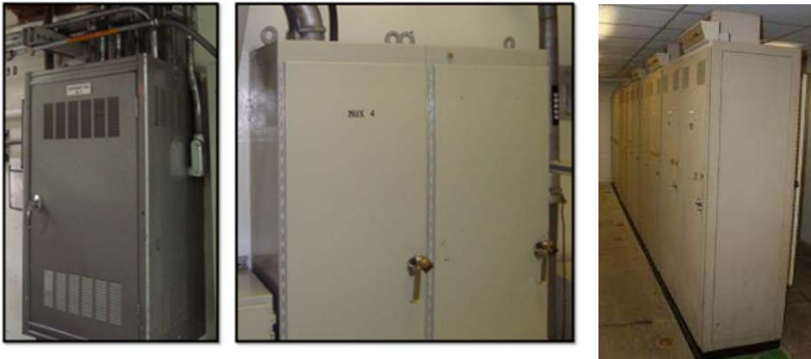
Figure C-21 Medium Enclosure (Approximately 2 ft. x 2 ft. x 7 ft.)
