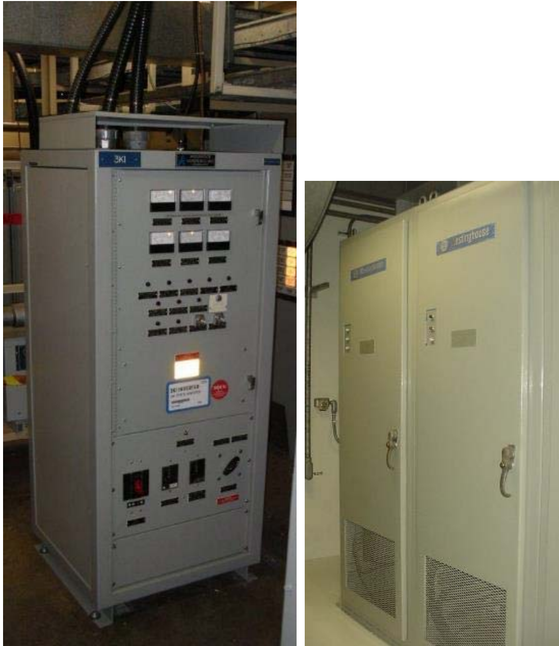
Figure 3-6 Examples of closed cabinets (a) fully closed cabinet and (b) closed with openings at the bottom
