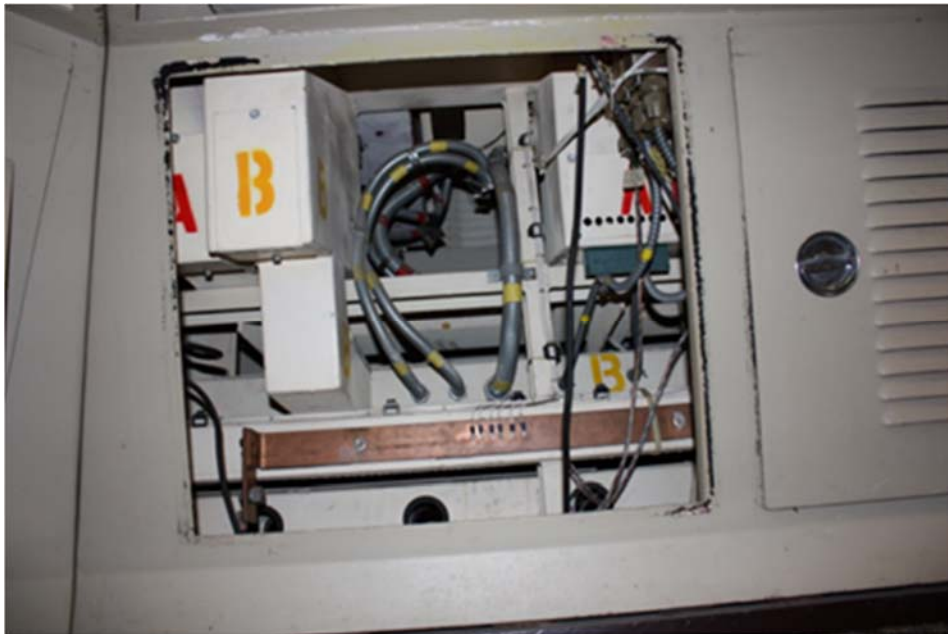
Figure 4-5 Photograph of Switch/Devices Cover (Labeled B) Within an Electrical Enclosure
