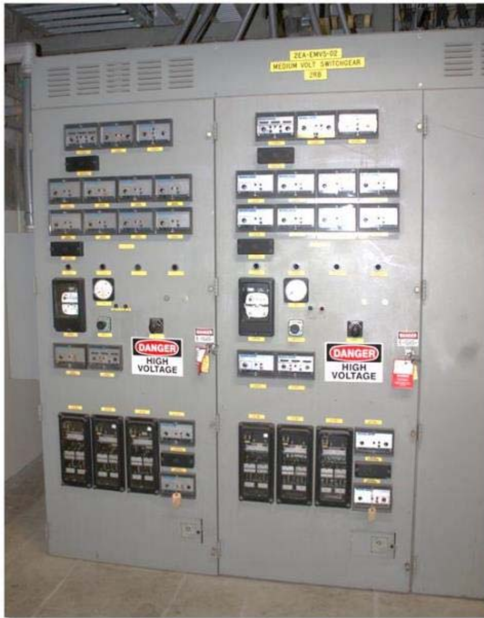
Figure C-2 Front View of 6.9 kV Switchgear Relay and Control Logic Enclosures
