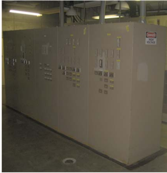
Figure C-17 Auxiliary Shutdown Panels – Large Enclosure (Closed)
