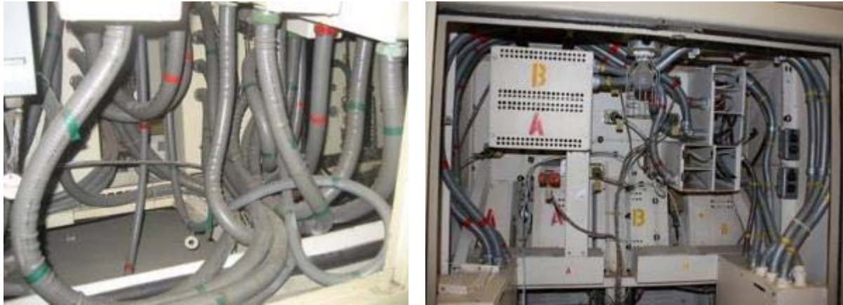
Figure 4-3 Photograph of LFMC (left) and FMC (right) Within Electrical Enclosure
