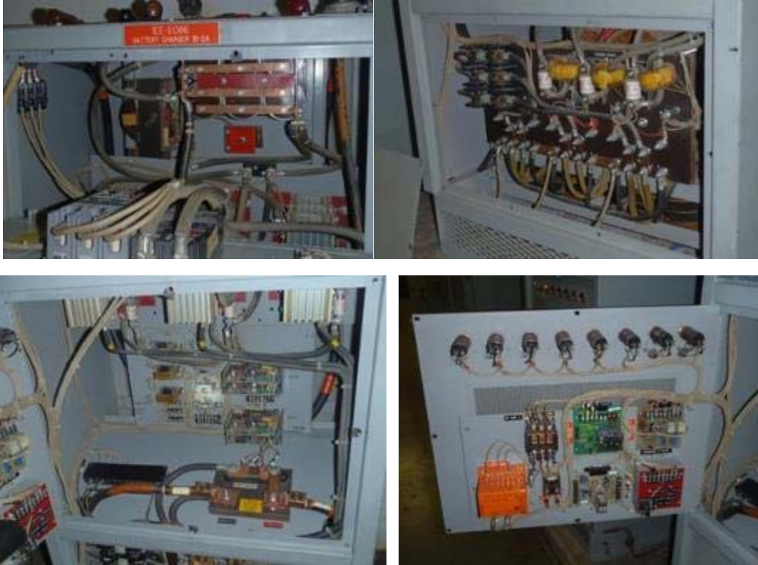
Figure C-14 Internal Views of Battery Chargers
