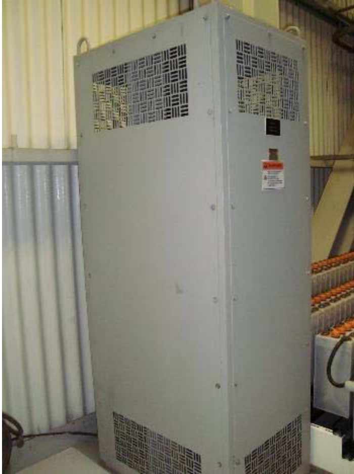
Figure 3-8 Example of closed cabinet with openings on the side panels at the top and bottom.
