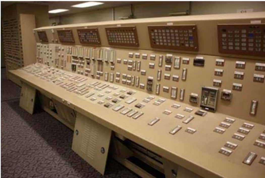
Figure C-19 Large Closed Electrical Enclosure (Main Control Board – MCB)
