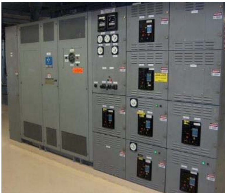
Figure C-8 Front View of Load Center (Right) and Transformer (Left)
