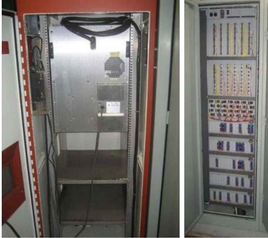
Figure 3-15 Two “Very Low Fuel Loading” Enclosures
