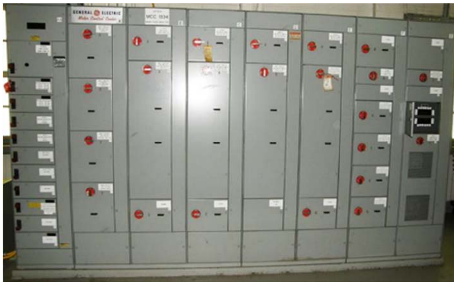
Figure 3-3 A Typical Bank of MCC Cabinets
