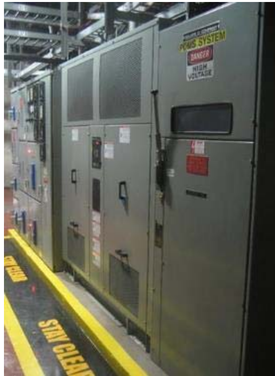
Figure C-5 Front View of Load Center (Disconnect Switch)
