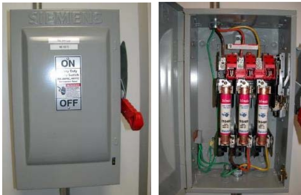
Figure C-23 Wall Mounted Low Voltage AC Fused Disconnect Switches
