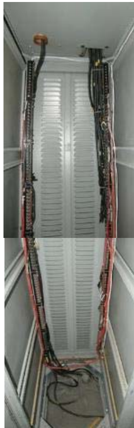
Figure 4-2 Cropped Photo of Electrical Enclosure with Bundled Panel Wiring and Cable, Limited Combustible Loading, and No Ignition Sources
