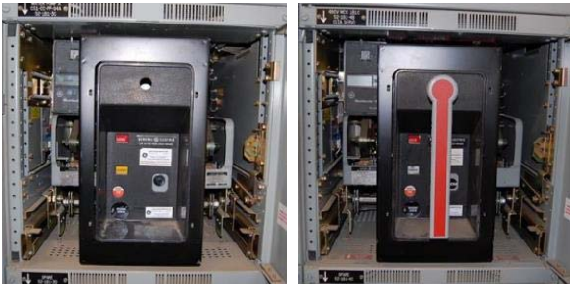
Figure C-10 Low Voltage Load Center Breaker
