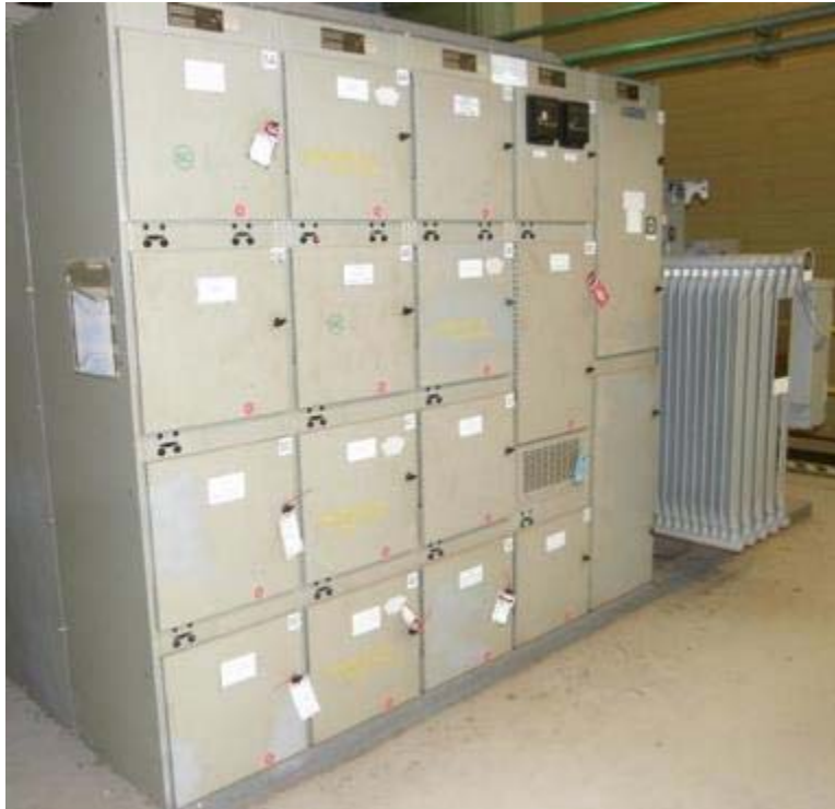
Figure C-7 Load Center (Left) with Oil-Cooled Transformer (Right)
