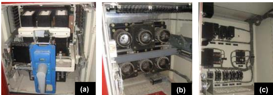
Figure C-6 Internal Views of a Load Center (a) Low Voltage Breaker, (b) Empty Breaker Cubicle, and (c) Load Center Control Cubicle
