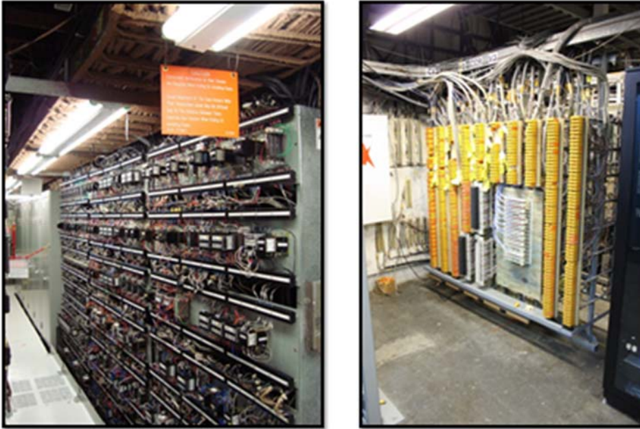
Figure 3-10 Additional examples of open cabinets
