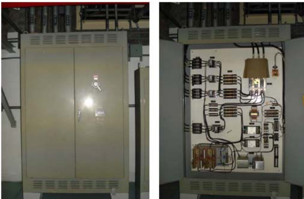
Figure 3-16 Large Enclosure (Closed and Open Configurations): Example of a “Low Fuel Loading” Subgroup
