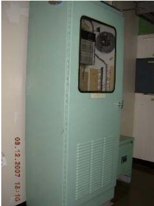
Figure 3-9 Example of an open cabinet with a combustible panel at top and louvers at the bottom of the front.
