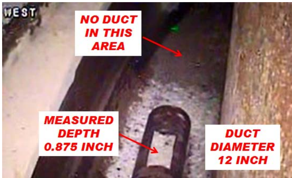
Figure 19: (Area at STA 8+00. Photo L U-ESR-H-00113)
