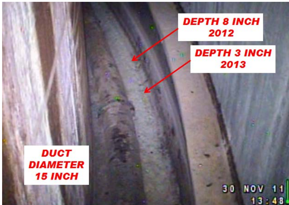
Figure 2: (Area at STA 5+00 estimated to a height of 8 inches in 2012. Attachment SRR-LWE-2012-00039)
