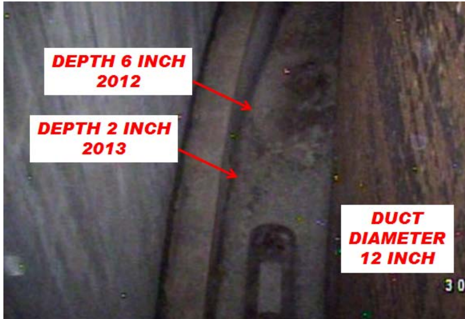
Figure 4: (Area at STA 8+00 interpolated to a height of 6 inches in 2012. Attachment SRR-LWE-2012-00039)
