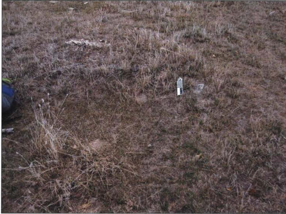
Figure 45. 25DW360 Feature F9, partial foundation, facing north. Photograph taken by Shane Rosenthal, on 11/20/2010.
