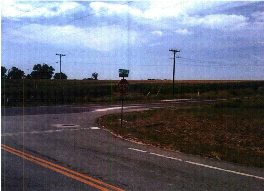
Figure 19-24. View of Proposed Radioisotope Production Facility Site from Intersection of New Haven and Rolling Hills Roads, Photo Location #7
