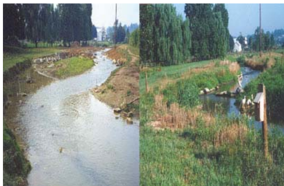
An eroding stream channel before (left) and after restoration (right).
