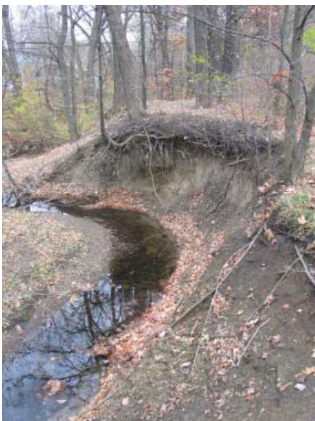
Severe erosion is common within the Dead River watershed.
