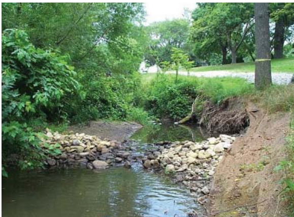
Artificial riffle installed in the downstream reach of Bull Creek to provide grade stabilization (BL07).
