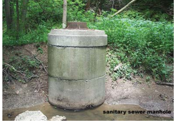
Exposed sanitary sewer manhole exposed by eroding streambank and streambed (BL08).
