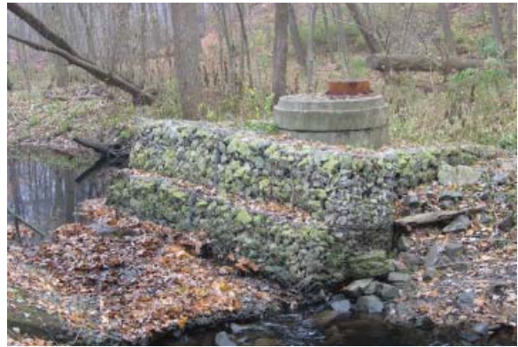
Structural, hard-edge protection for sewer infrastructure (BL08) protects the sewer but does not provide a natural stream habitat condition.
