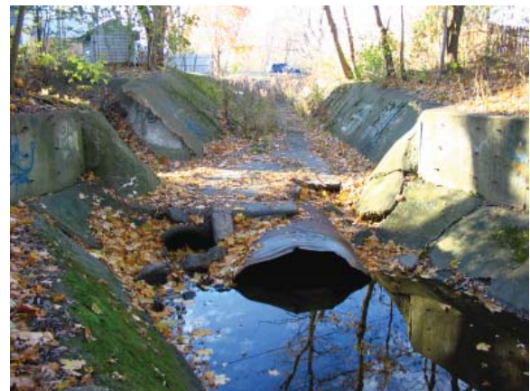
Severely impacted stream channel and armoring where reach BL15 crosses Wilson Street near Howard Street.
