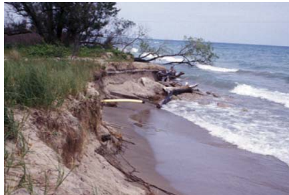
Beach erosion has exposed this buried pipe from 11 feet in 2003 to over 20 feet in 2005, Illinois Beach State Park
