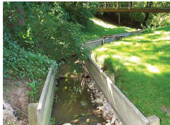
Armoring such as this wood retaining wall helps stabilize the streambanks but reduces the quality of the stream habitat for aquatic plants and animals (BL11).
