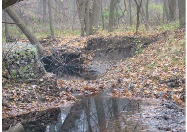
Erosion of the streambank opposite the sewer stabilization project (BL08).
