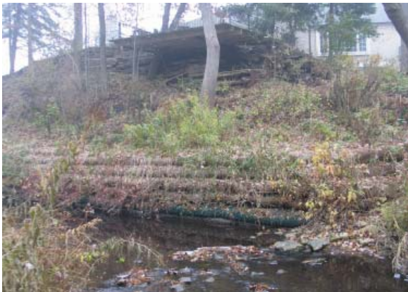
Soil lifts stabilizing the streambank, Bull Creek restoration project (BL07)
