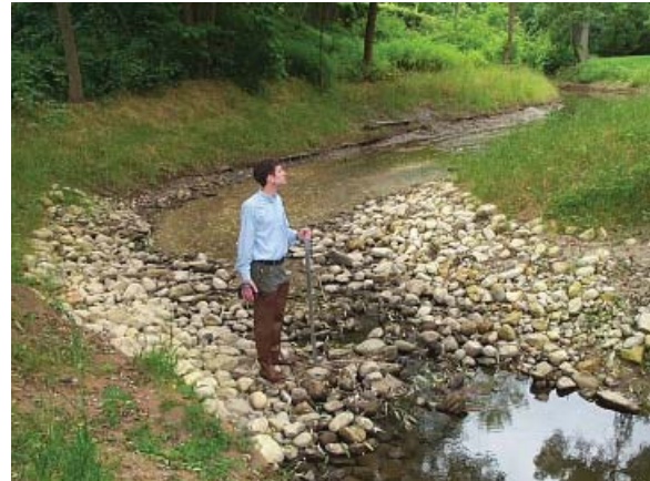
Rock riffle installed over exposed sanitary line to protect it.
