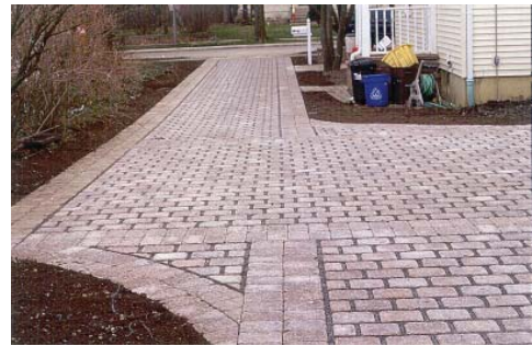
Porous Pavement (Elmhurst, IL)
