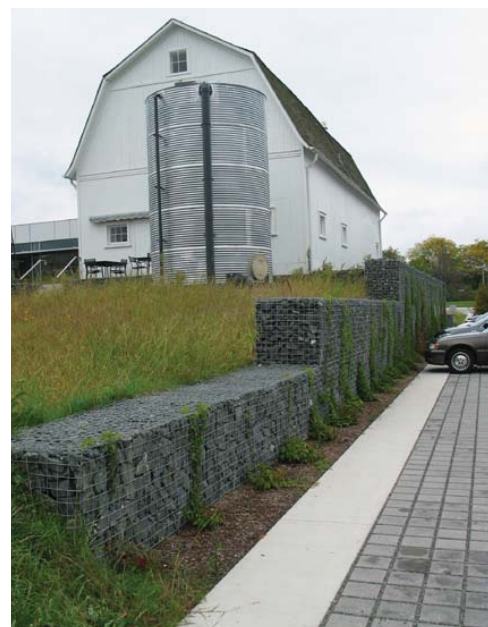
a cistern system collects rainwater from Kresge Foundation Headquarters (Toy, MI) (Photo: Conservation Design Forum)
