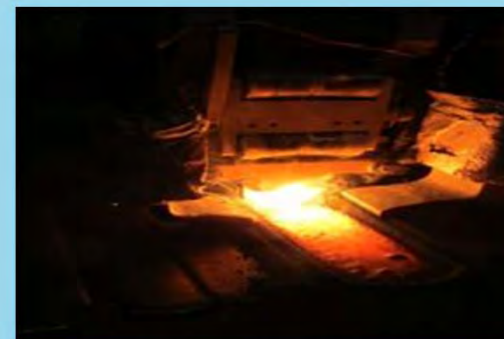
690 strip cladding mockups and process controls
