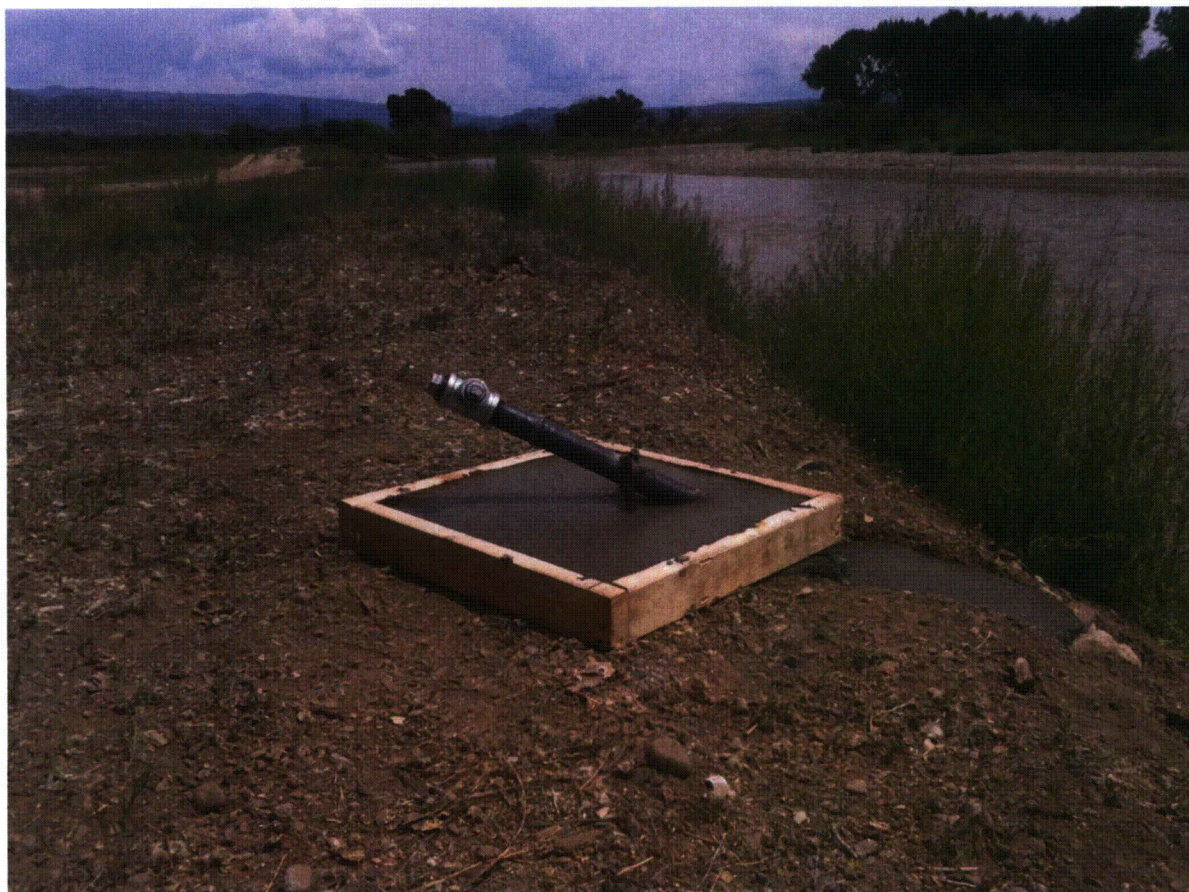
Figure 2. Example of Stilling Well Construction
