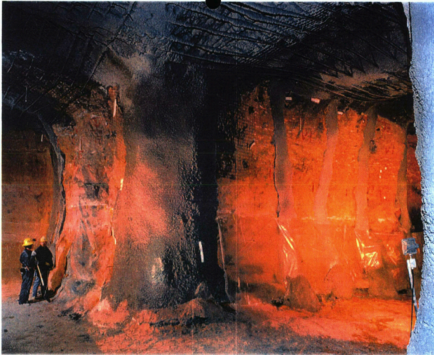
Final excavation of the test bed for the Unsaturated Zone Transport Test at Busted Butte.
