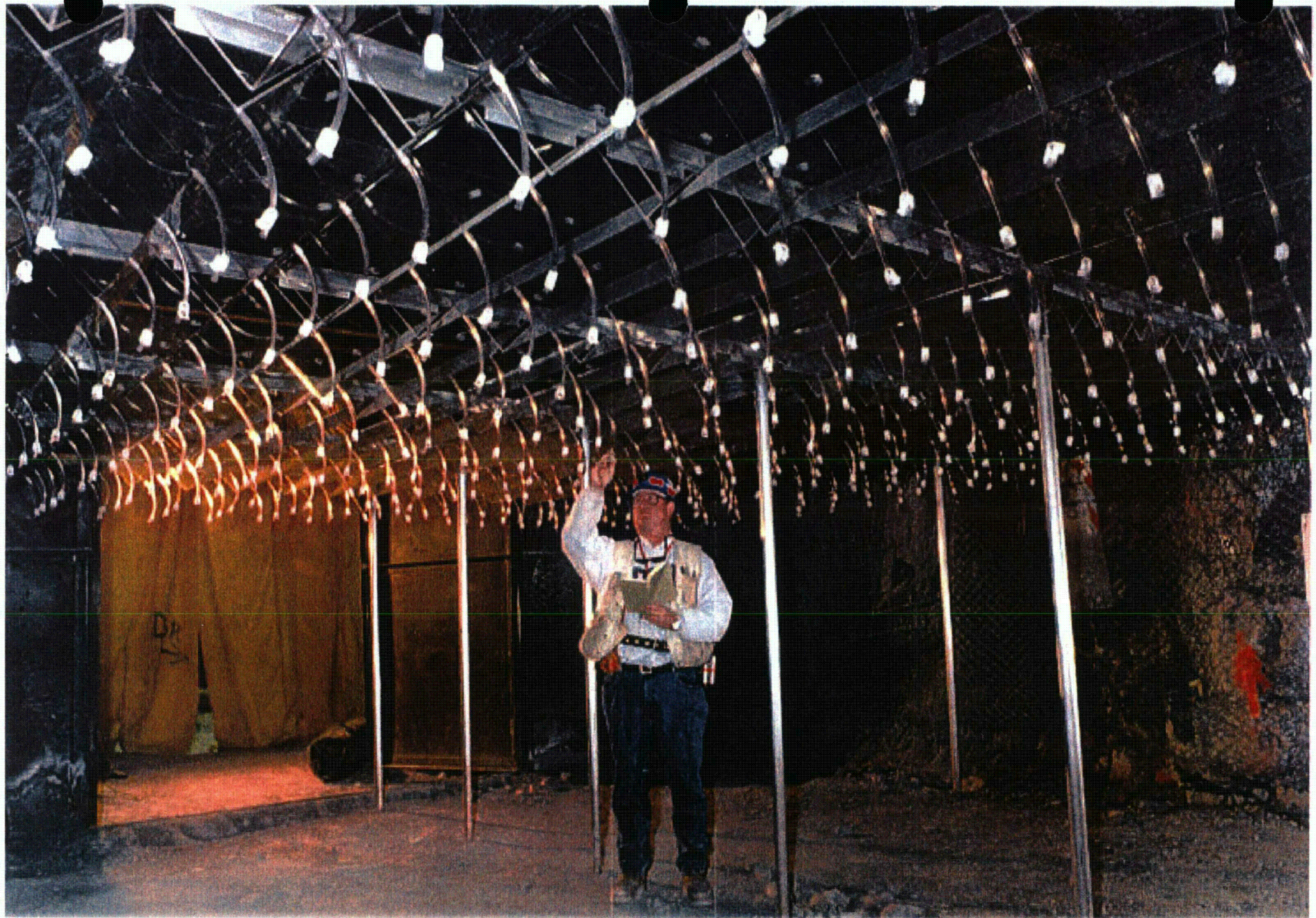
Collection trays installed on the roof of Alcove 1 to collect the water being released on top of Exile Hill.
