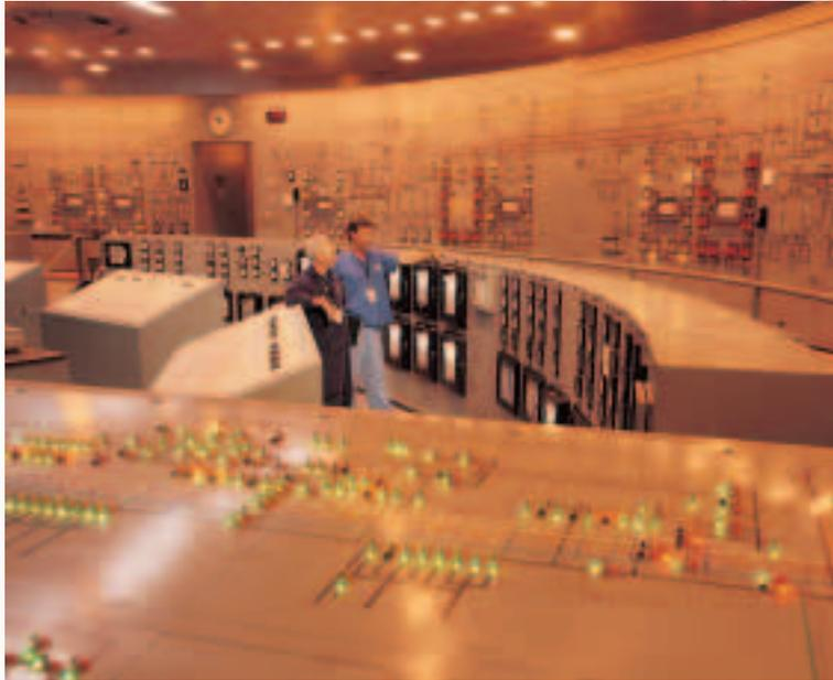
***The control room at the Paducah uranium enrichment plant is the center of all plant activity. From here, operators can monitor and control all enrichment operations on the plant site***
