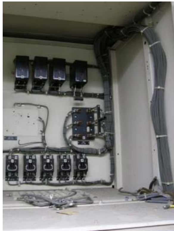
Figure 2-4. Photographs of the internal wiring of typical motor control centers.
