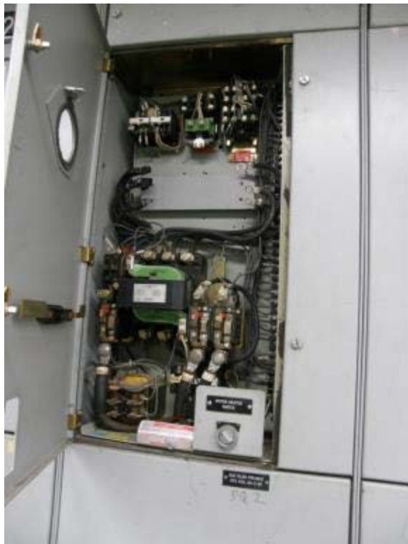
Figure 2-4. Photographs of the internal wiring of typical motor control centers.
