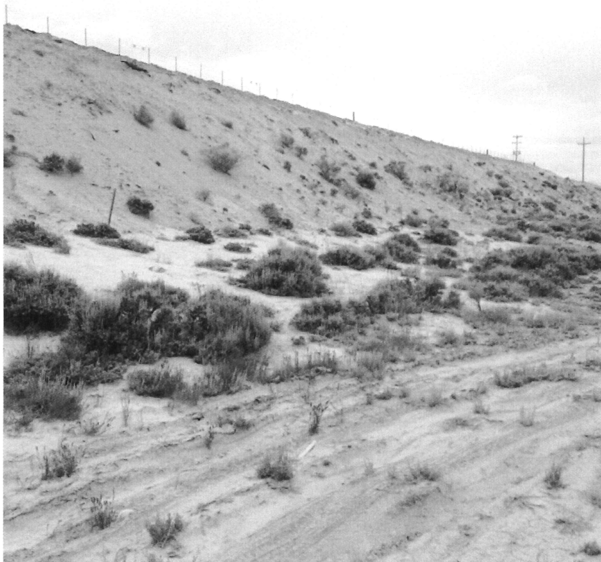
Photograph 1 Exterior of the west embankment.
