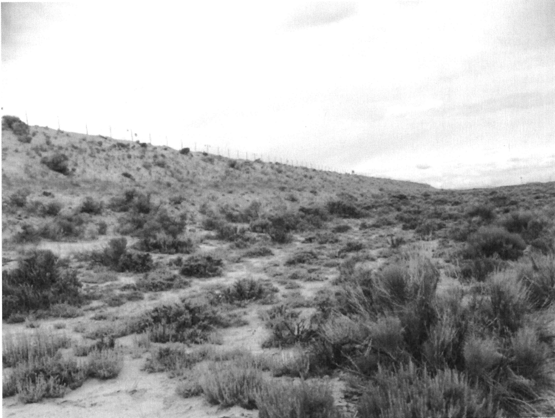
Photograph 4 Exterior of the north embankment.
