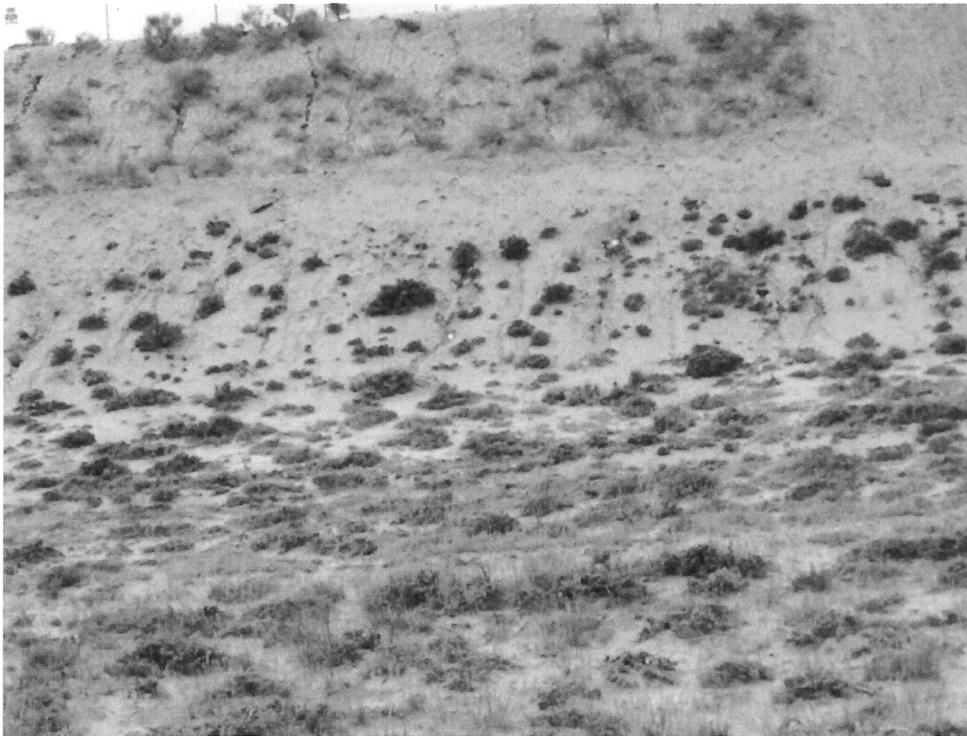
Photographs 3 Exterior of the east embankment, minor rills.
