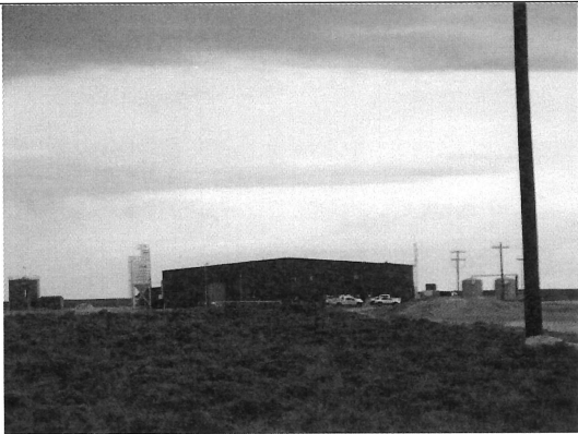
Image 1 – UR Energy Lost Creek Project Offices – May 29, 2014
