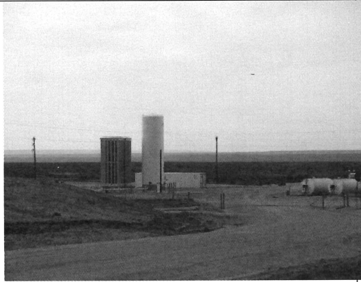
Image 2 – UR Energy Lost Creek Project Liquid Oxygen Tank – May 29, 2014
