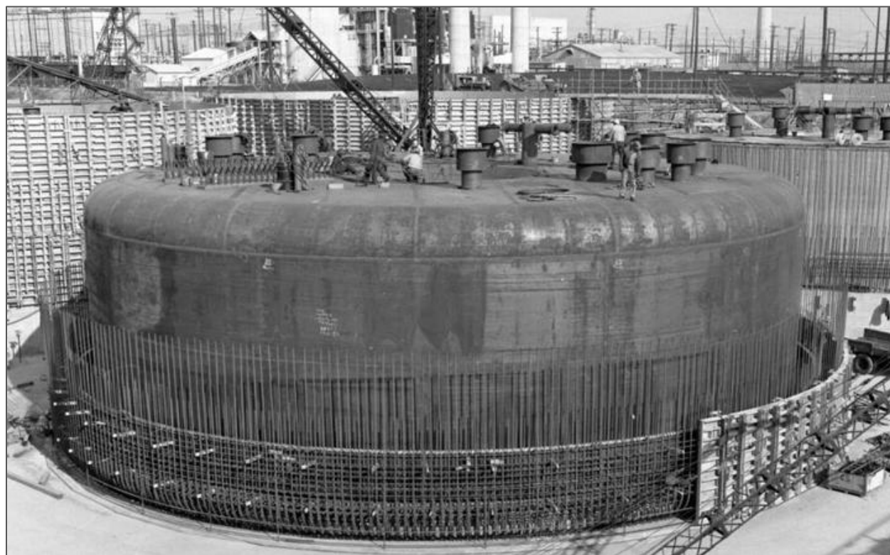
Figure 3.3-2: Type II Tank with Primary and Secondary Liner
