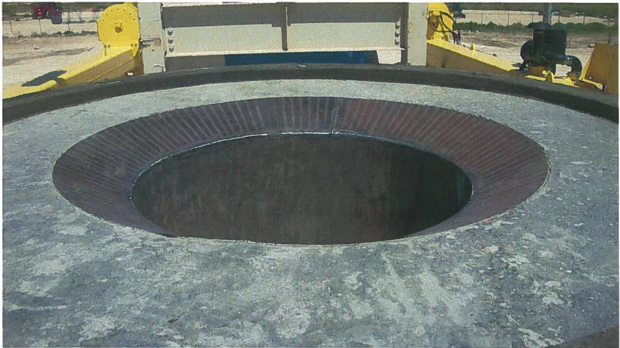
Figure 3, Modular Concrete Canister Used for Disposal of Irradiated Hardware.
