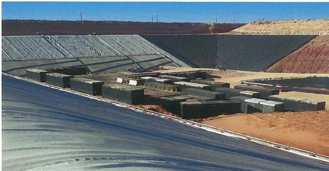
Figure 1, WCS Federal Waste Disposal Facility.
