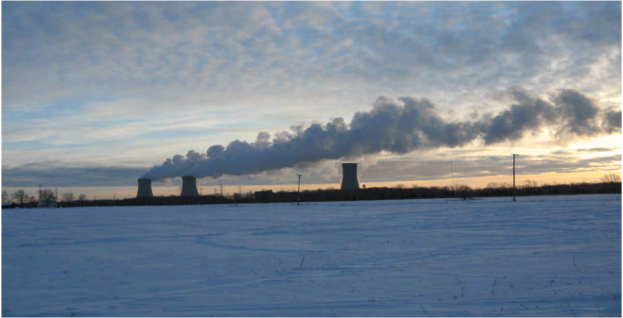
Figure 3.1-6 View of Fermi Site from Toll Road Looking East
