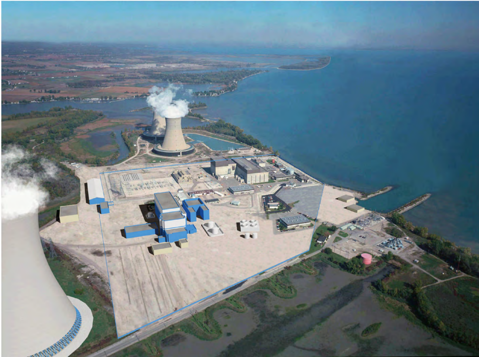
Figure 3.1-1 Aerial View of Fermi Site Looking North - Fermi 3 Superimposed
